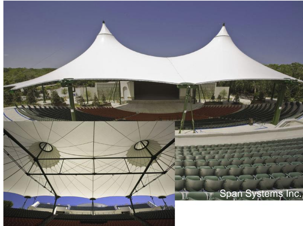
Tensioned membrane roof (St Augustine, Florida, USA)
