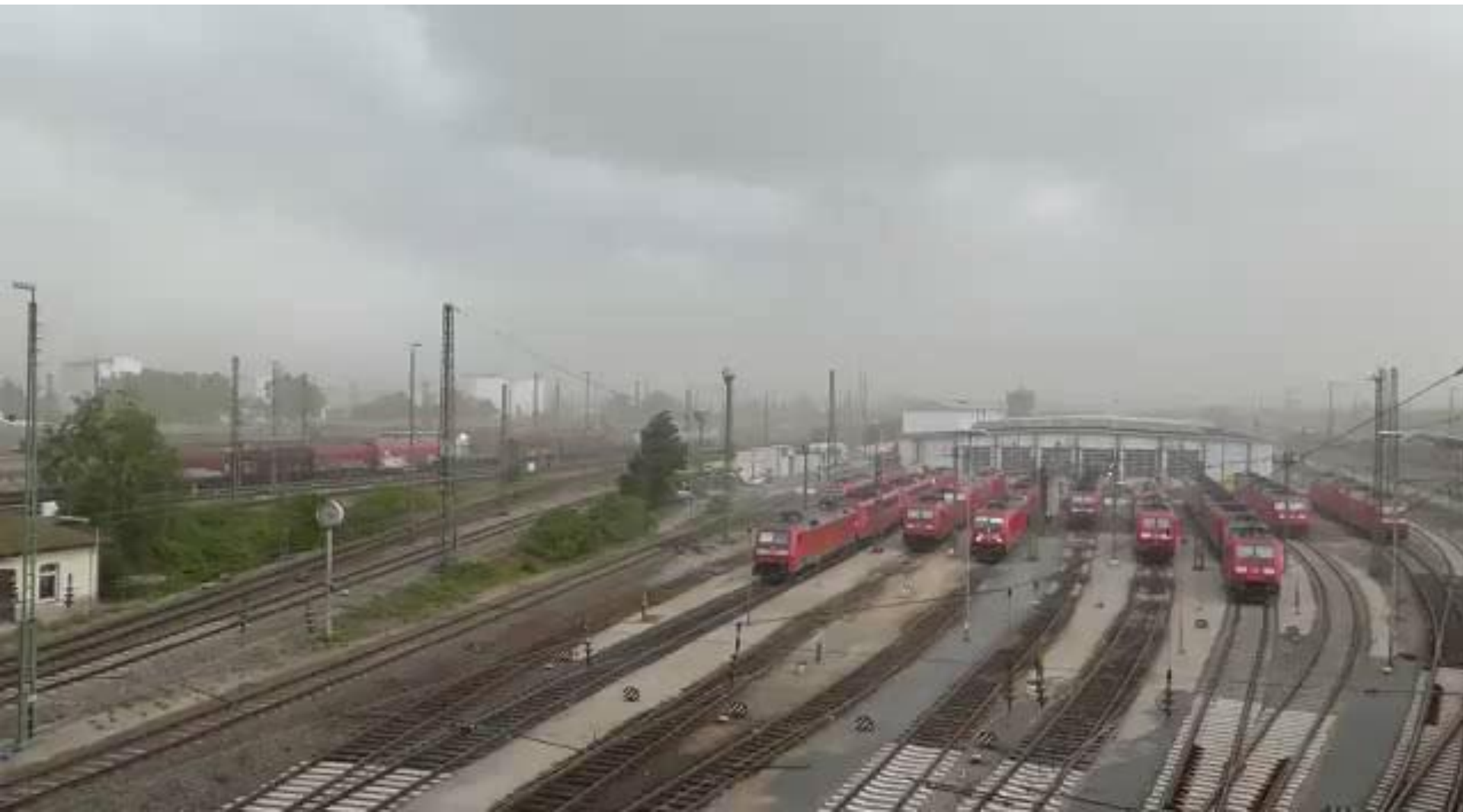
Wind damage, Mannheim train shed 9th August, 2018
