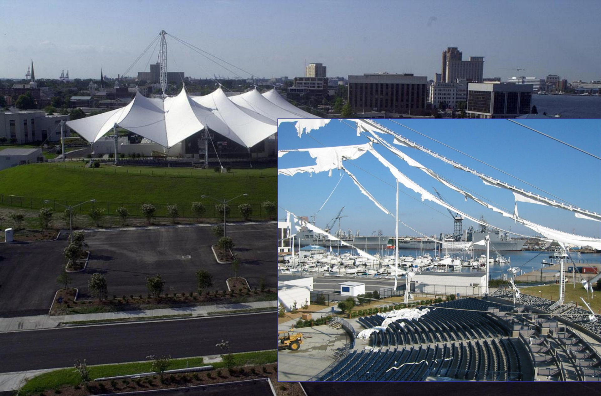
Open air theatre damaged during a hurricane (Portsmouth, Virginia, USA)
